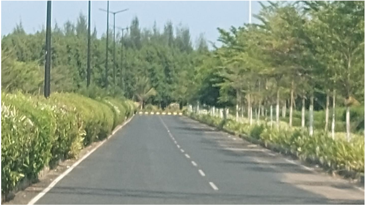
GREEN COVER ALONG PIPE RACK & INTERNAL ROADS
