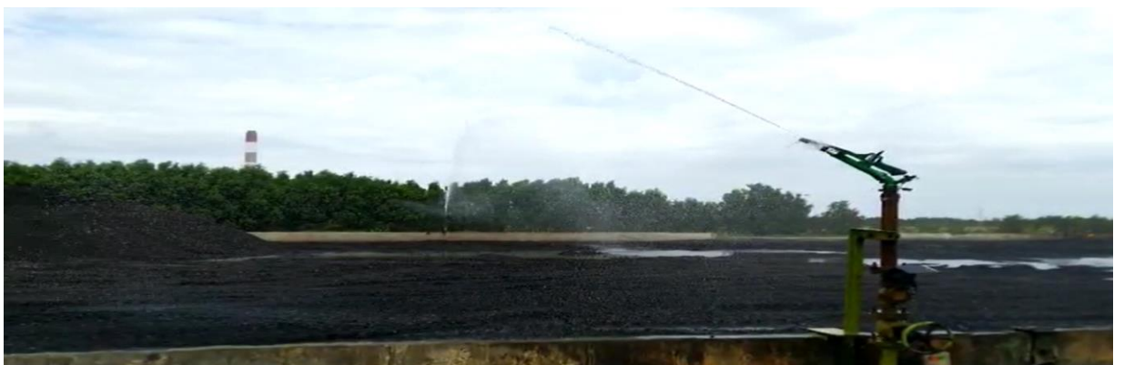
COAL YARD WATER SPRINKLING
