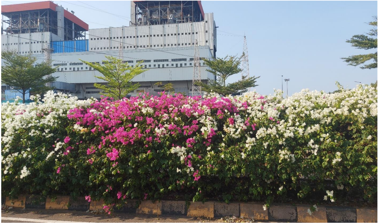
GREEN COVER NEAR PLANT SERVICE BUILDING
